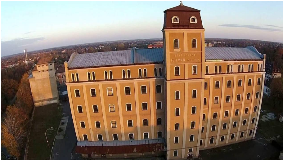
Figure 2 - The mill before the fire 18
