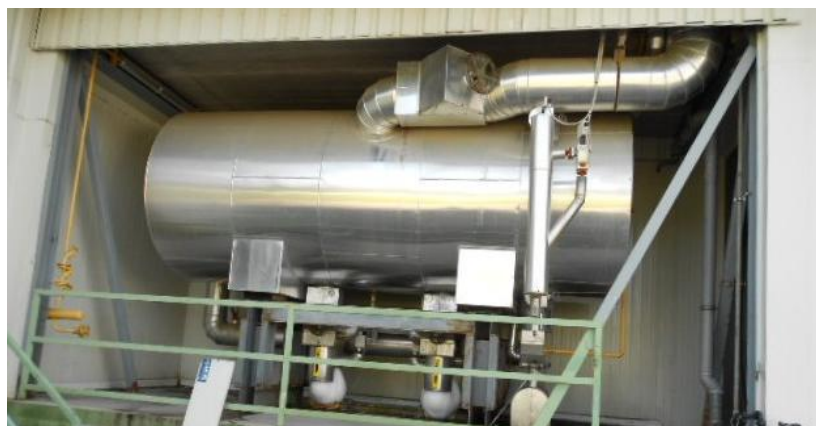
Figure 1. Ammonia tank (directly next to the neighboring dwelling-house)
