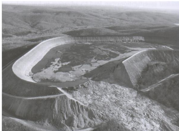
Figure 6. Failure of Taum Sauk reservoir (photograph courtesy of Ameren)
