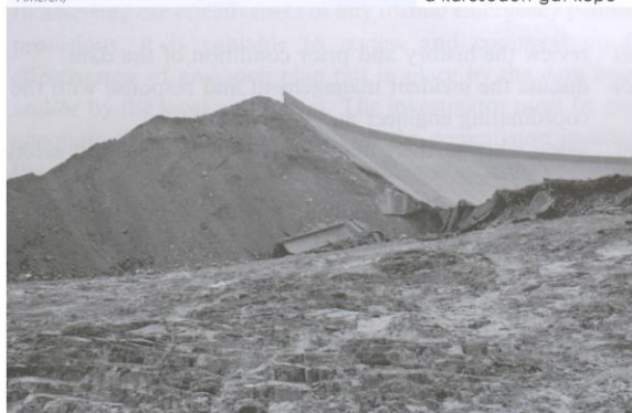
Figure 6. Failure of Taum Sauk reservoir (photograph courtesy of Ameren)
